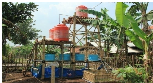
Figure 1. Design of the biofilter reactor
