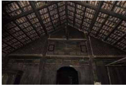
The partition of Oknha Baurtes Osman's house goes up to the roof.
