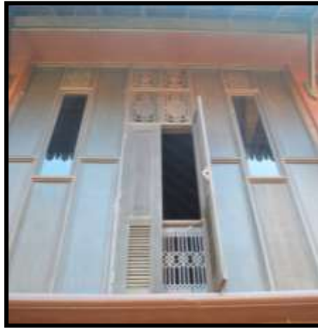
Picture 5: Carvings decorating doors for air and light distribution into the mosque
