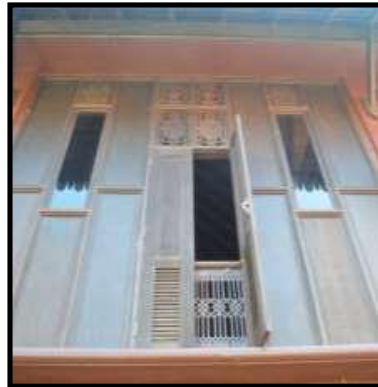
Picture 5: Carvings decorating doors for air and light distribution into the mosque
