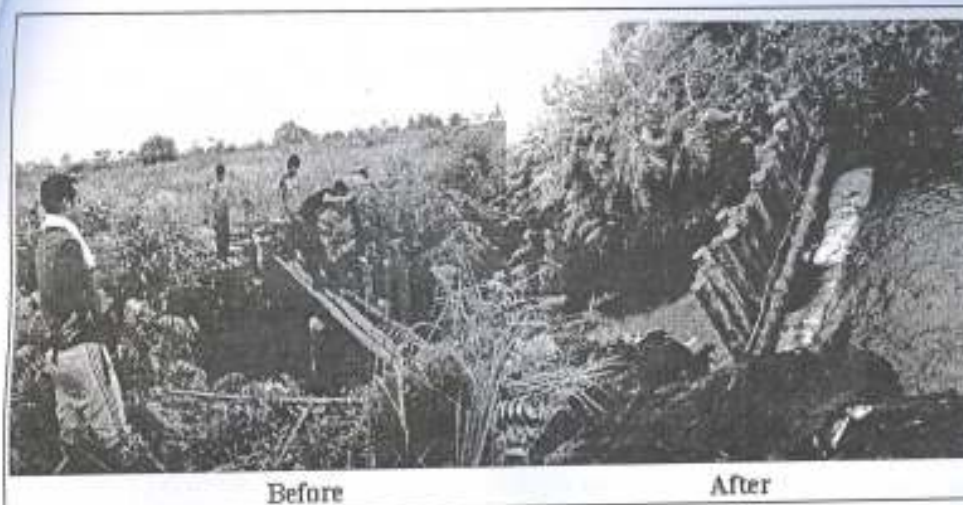
Figure 7. Establishing simple block canal in Tanjung Leban Village.
