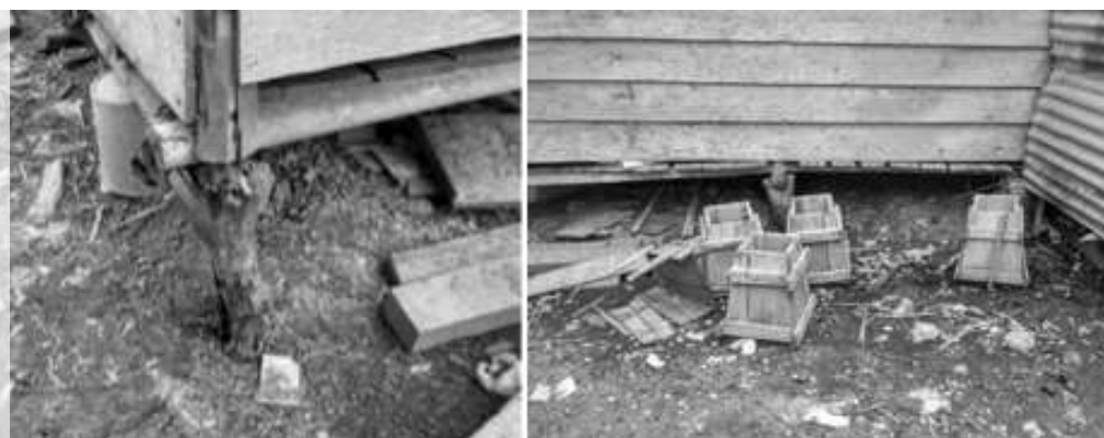
Figure 4. Replacing house's pile to concrete pedestal
