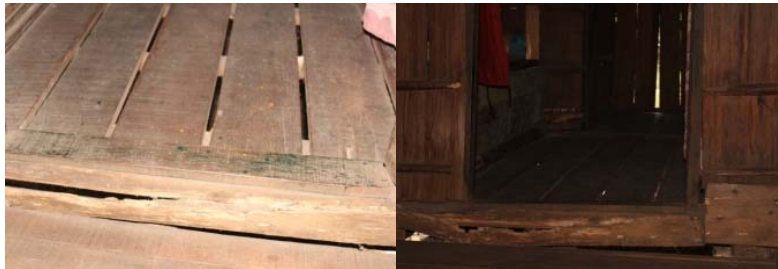
Figure 13. Bendul on the floor as divider the space Source: Survey, 2014
