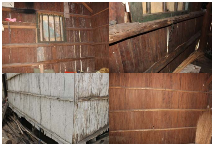
Figure 10. Sinto (above) and pengapit (below) on Lum's House Source: Survey, 2014
