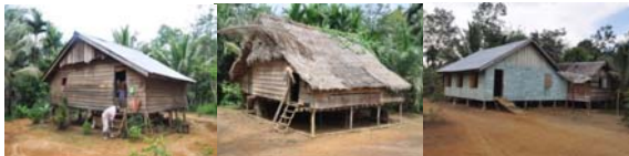
Fig.8. Variation of Material Application on Talang Mamak Tribe's House : Zinc (left), Leaves (Center), and Combination of Leaves and Zinc (Right) Source: Faisal, 2013
