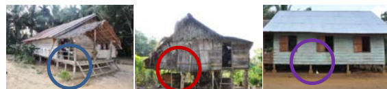
Fig.12. Pillars Form of Talang Mamak Tribe's House Source: Faisal, 2013
