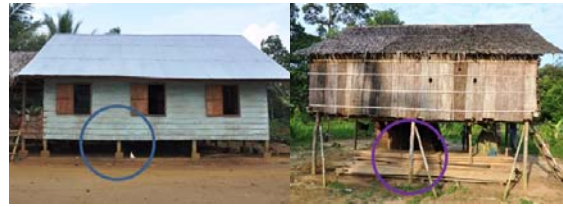
Fig.14. Variation of Detail Pillars Material Application on Talang Mamak Tribe's House Source: Faisal, 2013
