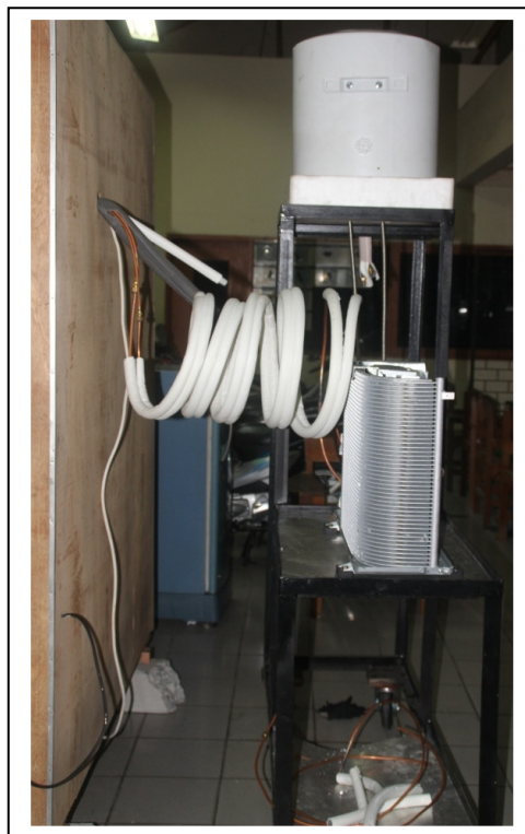
Gambar L2.10. Proses instalasi Sistem Refrigerasi tampak samping sisi outdoor
