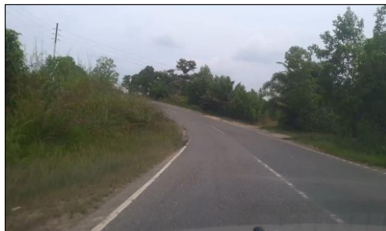
Figure 8. The vertical bends within the existing highway locations at KM 44 + 95.
