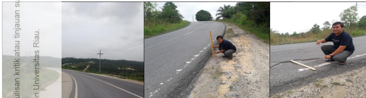
Figure 3. (a) Sharp turnings (bends) without traffic signs and no streetlights, (b) the existing highway condition with no road shoulder and no streetlights, (c) the existing patching holes. Source: Survey data, 2015.
